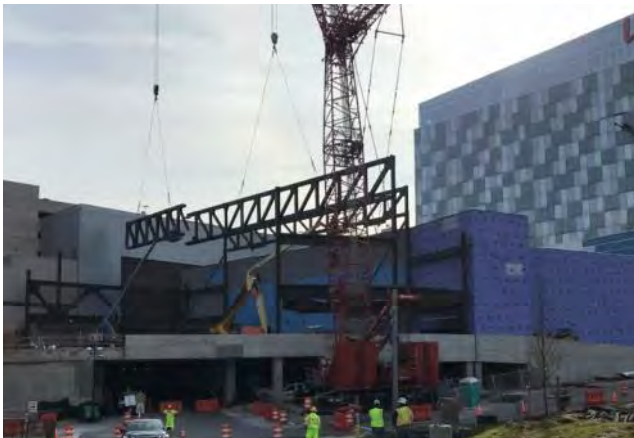
THE HALL AT LIVE! TRUSS ERECTION SEQUENCING AND LOGISTICS
