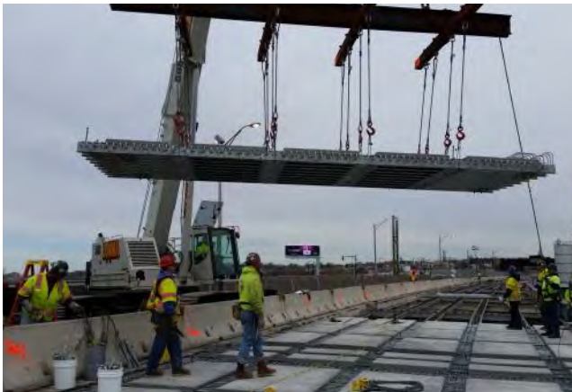
PULASKI SKYWAY EXODERMIC PANEL RIGGING
