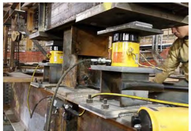
BOWTIE TEMPORARY SHORING, COLUMN LOAD TRANSFERS & CONSTRUCTION SEQUENCING
