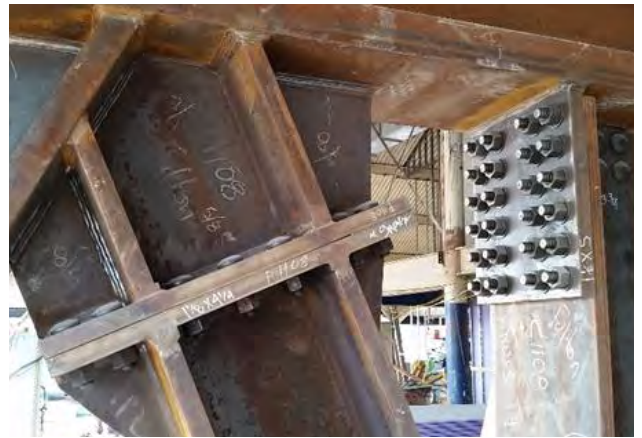
FIELD BOLTED CONNECTIONS
