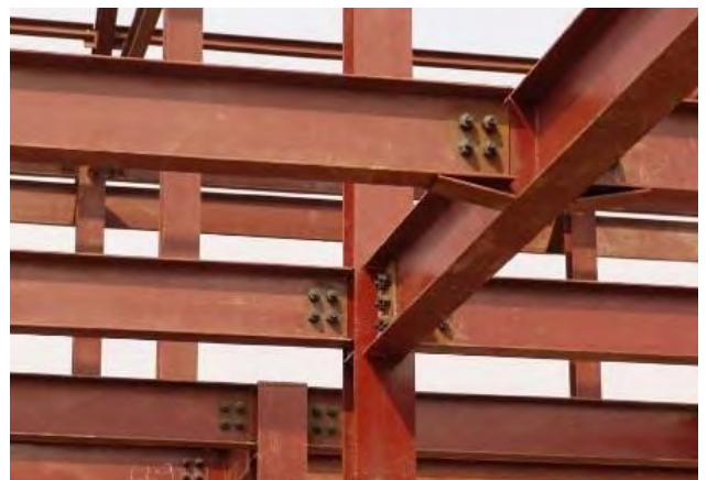
STANDARD SHEAR CONNECTIONS
