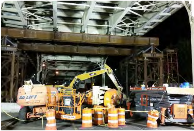
MACOMBS DAM BRIDGE TEMPORARY SHORING & JACKING
