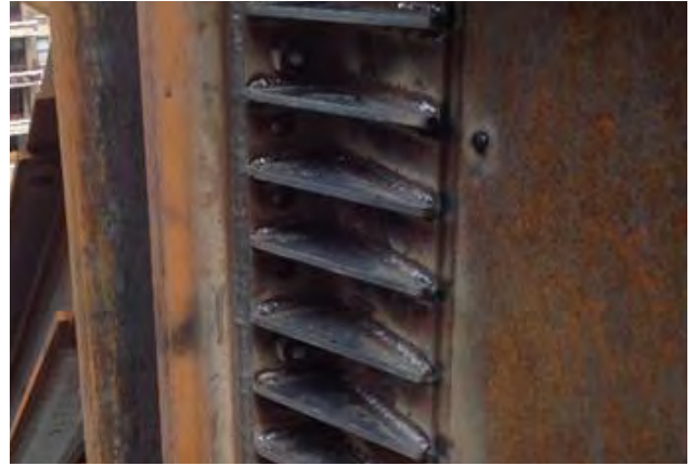
REINFORCEMENT OF EXISTING CONNECTIONS
