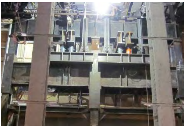
JACKING & REMOVAL OF COLUMN TRANSFER GIRDER FOR 1,000,000 LB LOAD
