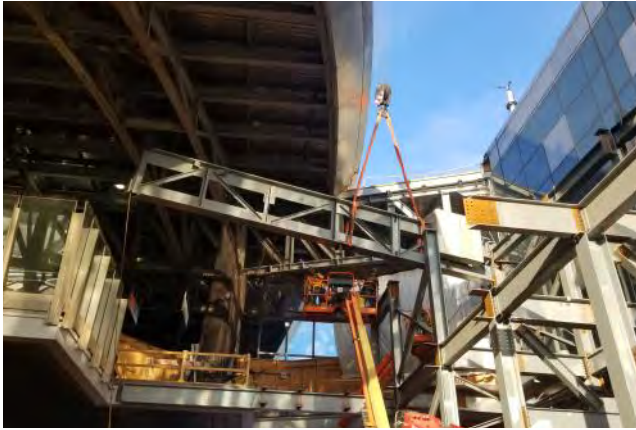
JAMAICA STATION COUNTERWEIGHT TRUSS RIGGING
