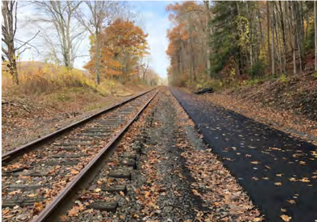
MAYBROOK TRAILWAY DESIGN-BUILD
