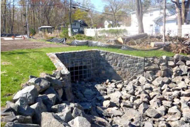
QUASPECK PARK DRAINAGE IMPROVEMENTS
