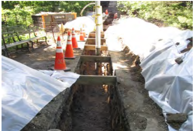
GEO THERMAL DRILLING
