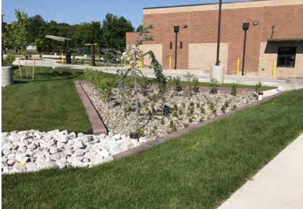
STORMWATER MANAGEMENT FACILITIES
