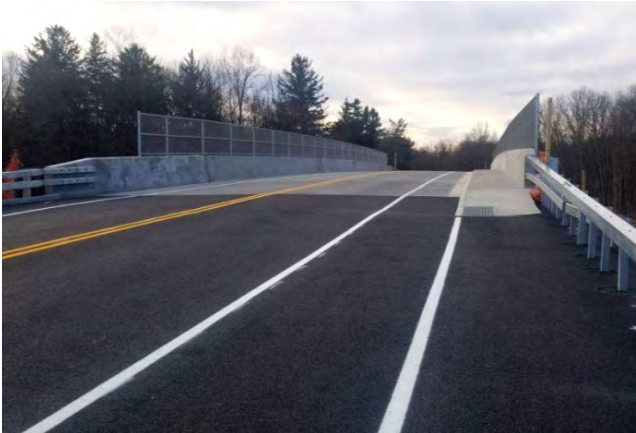
HUNGRY HOLLOW BRIDGE REPLACEMENT
