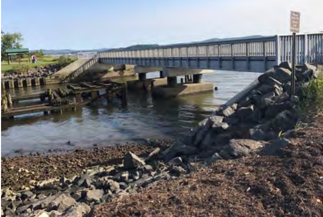
HAVERSTRAW COUNTY PARK RECYCLED PLASTIC BRIDGE
