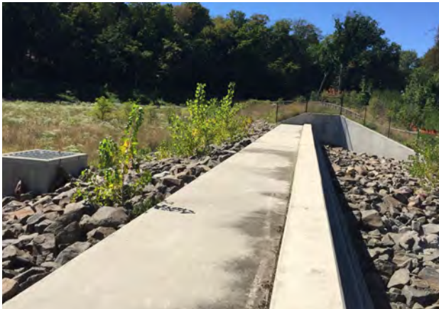
CENTRAL NYACK DAM
