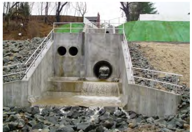
LIRR AMOTT DRAINAGE CULVERT REHAB
